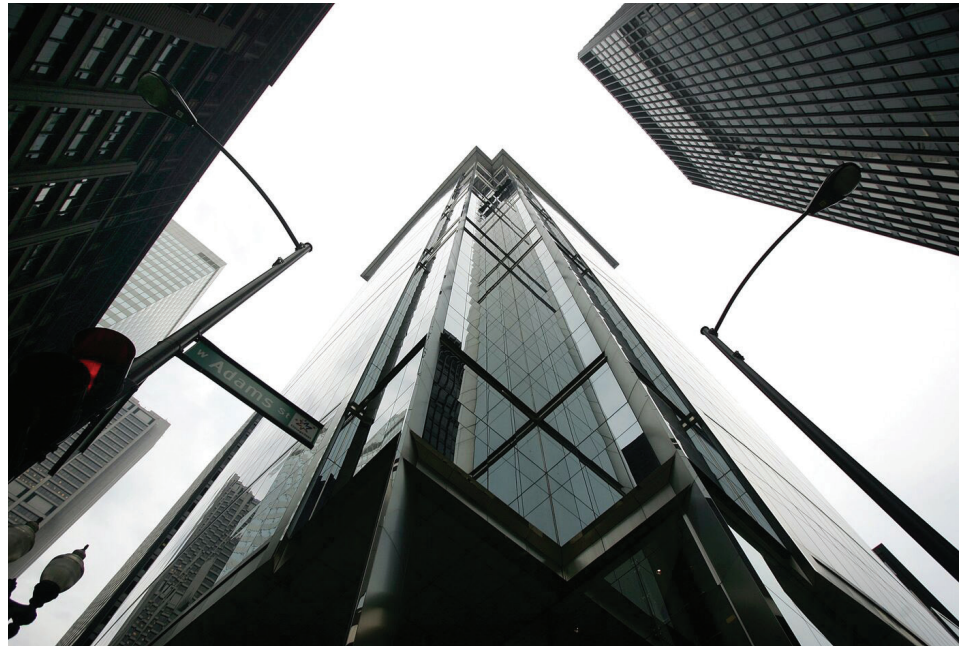
The building that houses Citadel Securities in Chicago Photographer: Tim Boyle/Bloomberg
